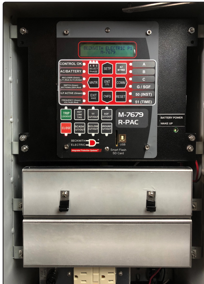
Figure 42 M-2406 Chassis Fully Installed
