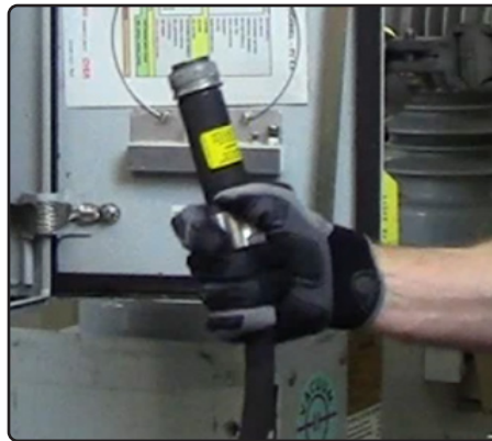
Figure 2 Disconnect 14-, 19-, or 26-Pin Recloser Cable
