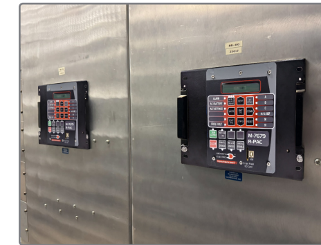
Figure 7 M-2406, Panel-Mount Application Example
