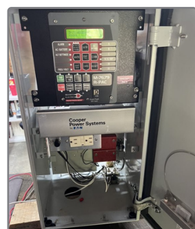
Figure 5 M-2406, Yard-Mount Application Example
